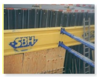
The application is very easy also in narrow site conditions: The excavator is located in front of the trench and lowers the trench sheets following the excavation with the excavator bucket. Alternatively the lowering can take place by means of ramming equipment.
