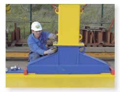
Depending on the trench width, flange the strut extensions onto the rolling struts.
