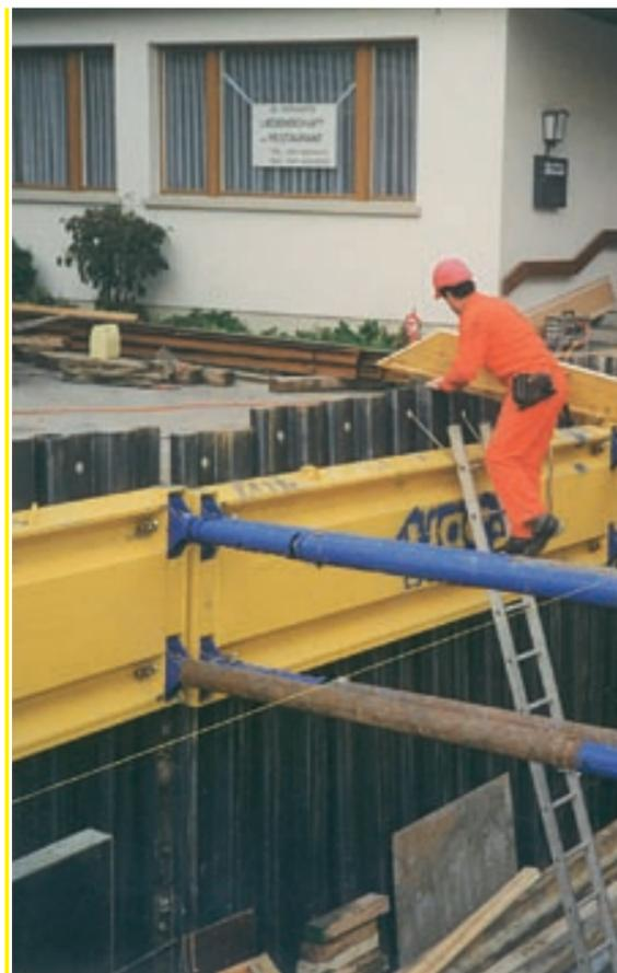
Pile chamber plates can be combined with any other SBH shoring system even with the SBH Rolling strut shoring system.
