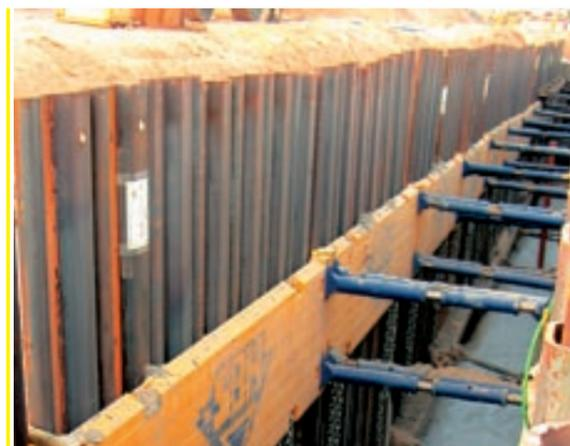
The pile chamber is produced for the trench sheet type KD 6/8. Larger trench depths require additional supports. The SBH Design Calculation Department offers professional advice and on request a design calculation especially for your site is provided.
