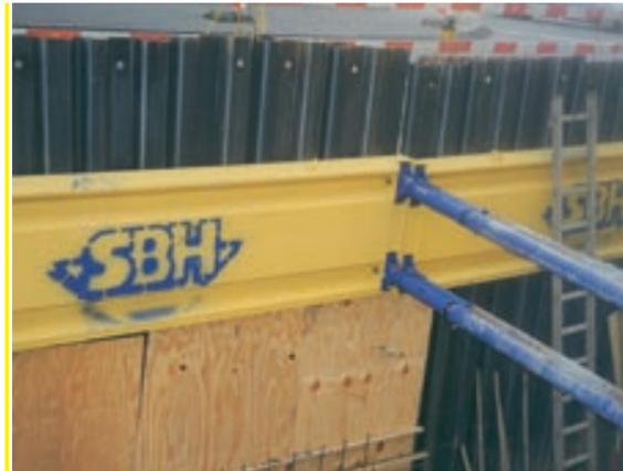
The application is very easy also in narrow site conditions: The excavator is located in front of the trench and lowers the trench sheets following the excavation with the excavator bucket. Alternatively the lowering can take place by means of ramming equipment.
